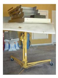
2. Position One-Touch underneath the ceiling rough opening.
