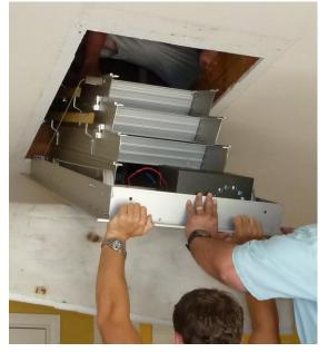
5. Once the overhanging portion of One-Touch is inserted into the opening, the operator of the tool can continue to raise One-Touch until its supporting structure is resting against the ceiling.
